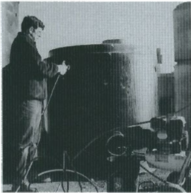
Power-spraying a coating of PPS 922 onto concrete.
